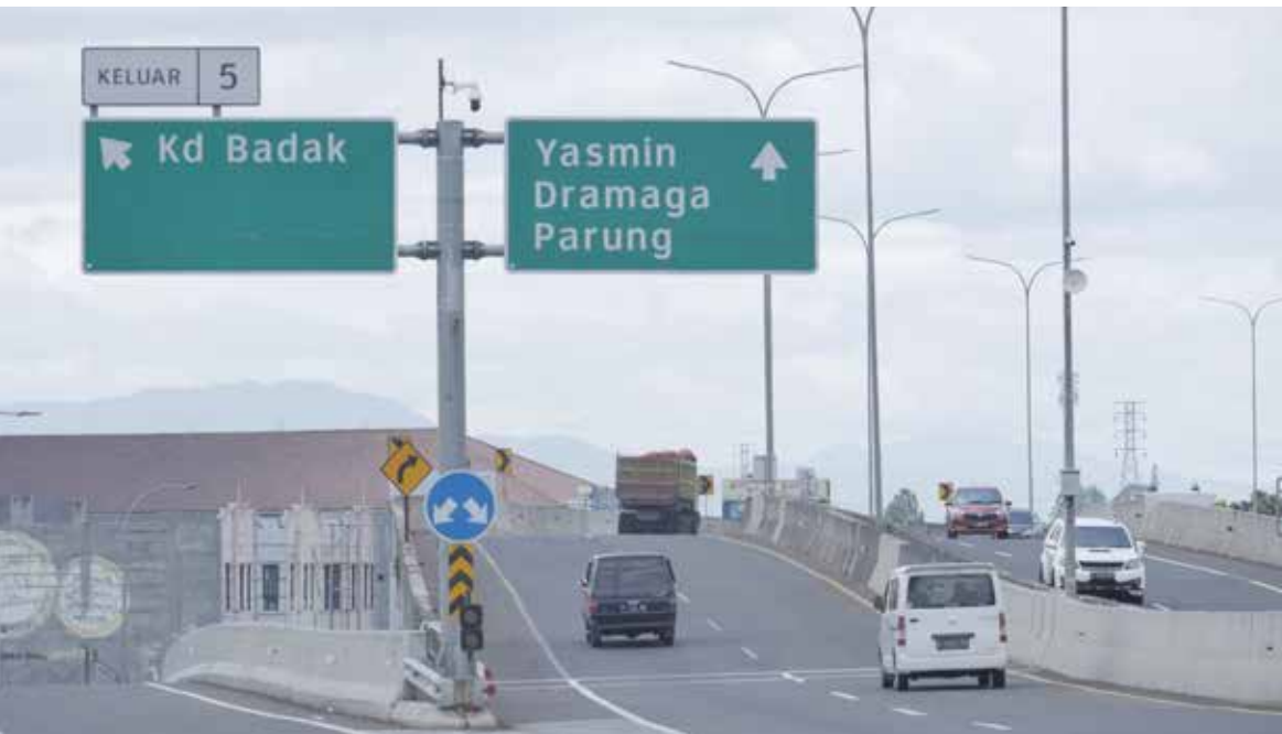
Jalan Tol Bogor Ring Road (BORR) Seksi 3A Ruas Simping Yasmin-Simpang Semplak
