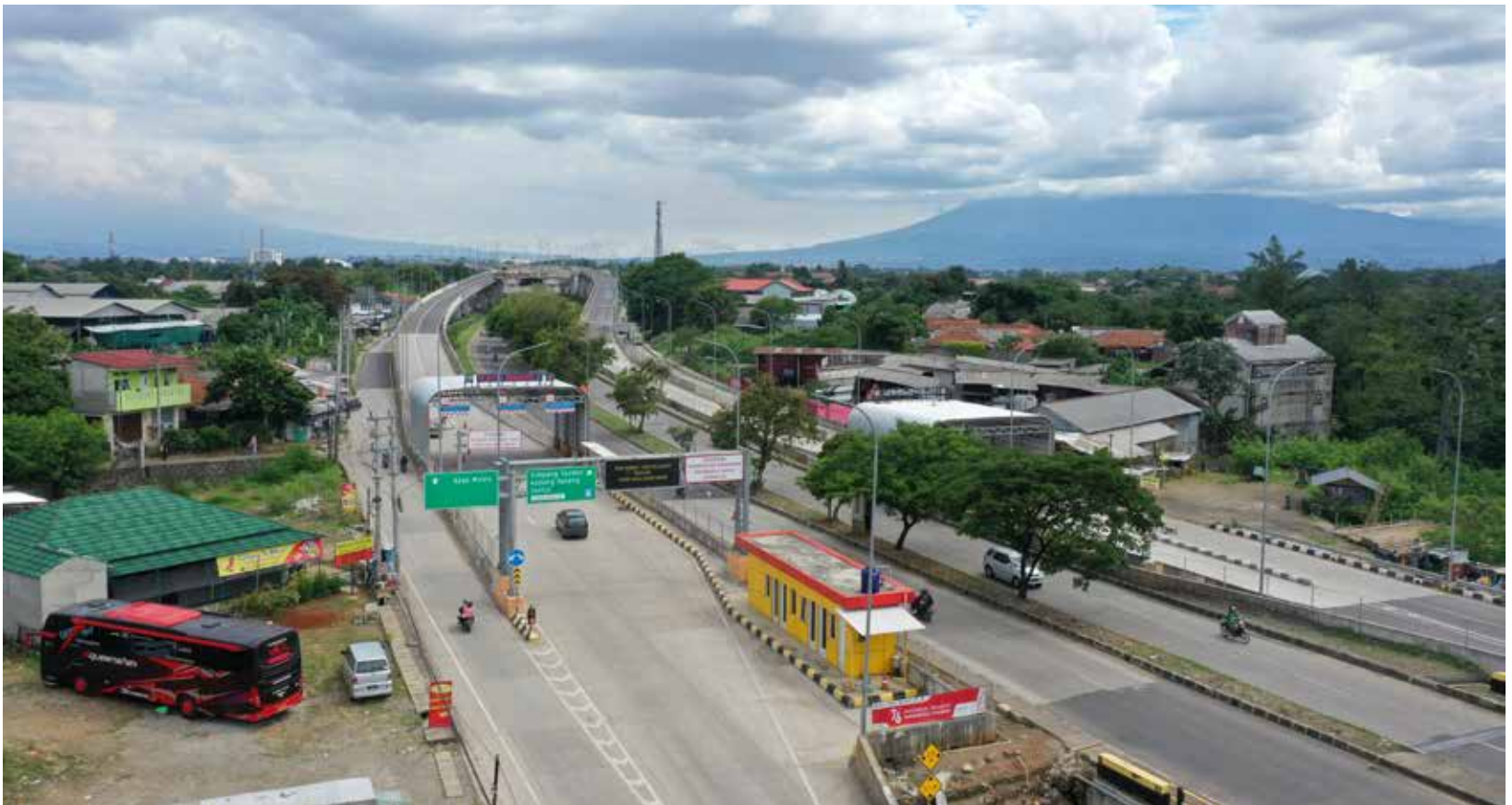
Jalan Tol Bogor Ring Road (BORR)
