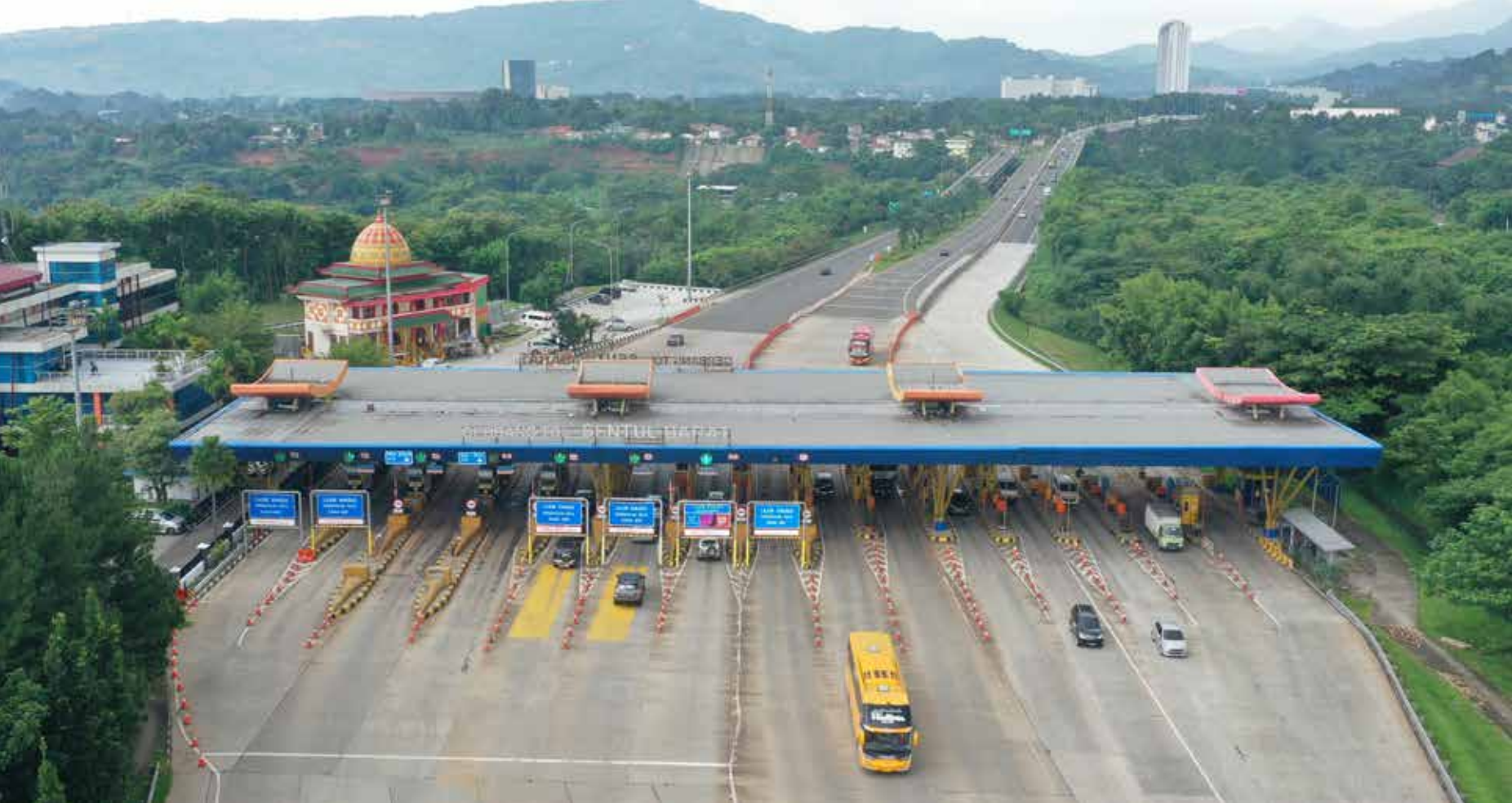
Gerbang Tol Sentul Barat Jalan Tol Bogor Ring Road (BORR)
