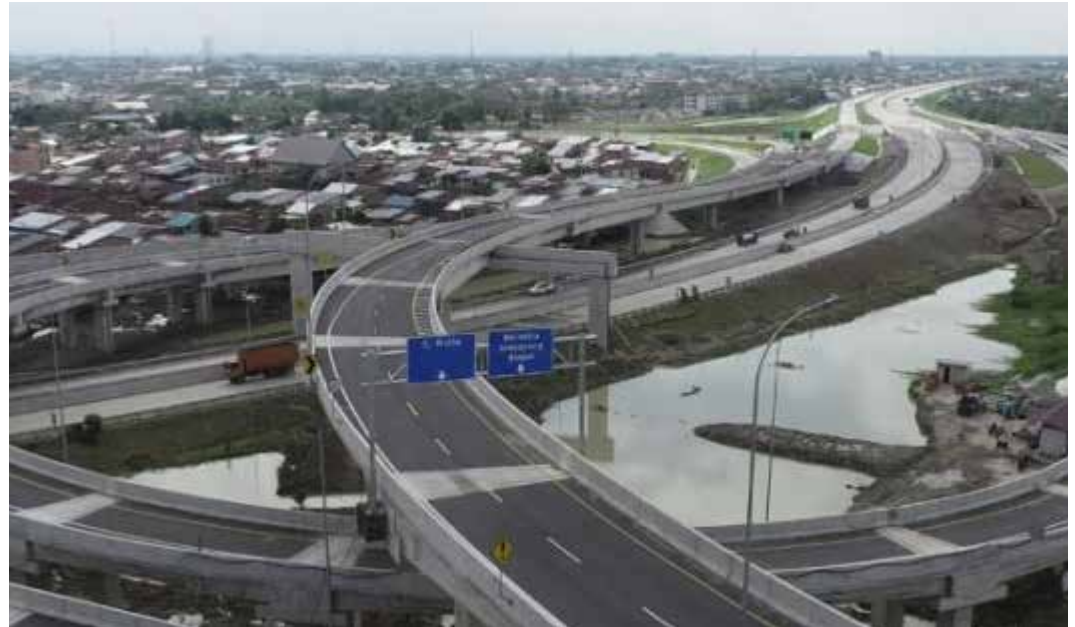
Jalan Tol Medan-Binjai Seksi 1 Segmen Junction Tanjung Mulia-Marelan
