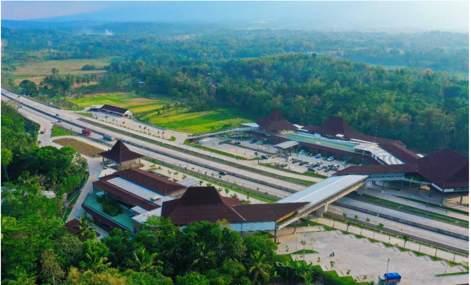
Rest Area Km 456 Skybridge Jalan Tol Semarang - Solo
