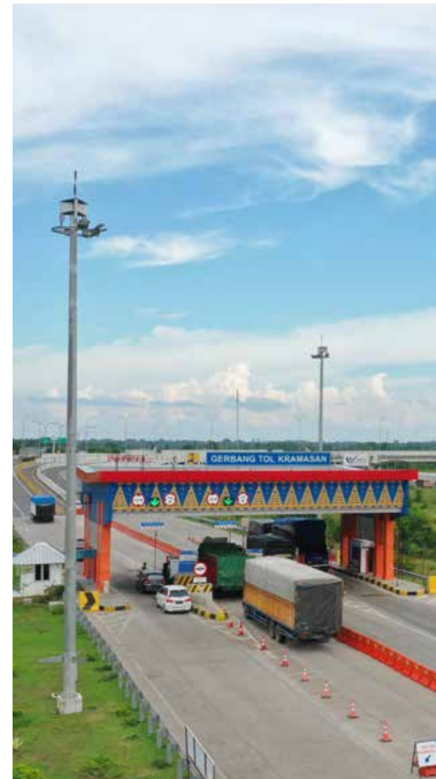
Gerbang Tol Keramasan Jalan Tol Kayu Agung-Kramasan
