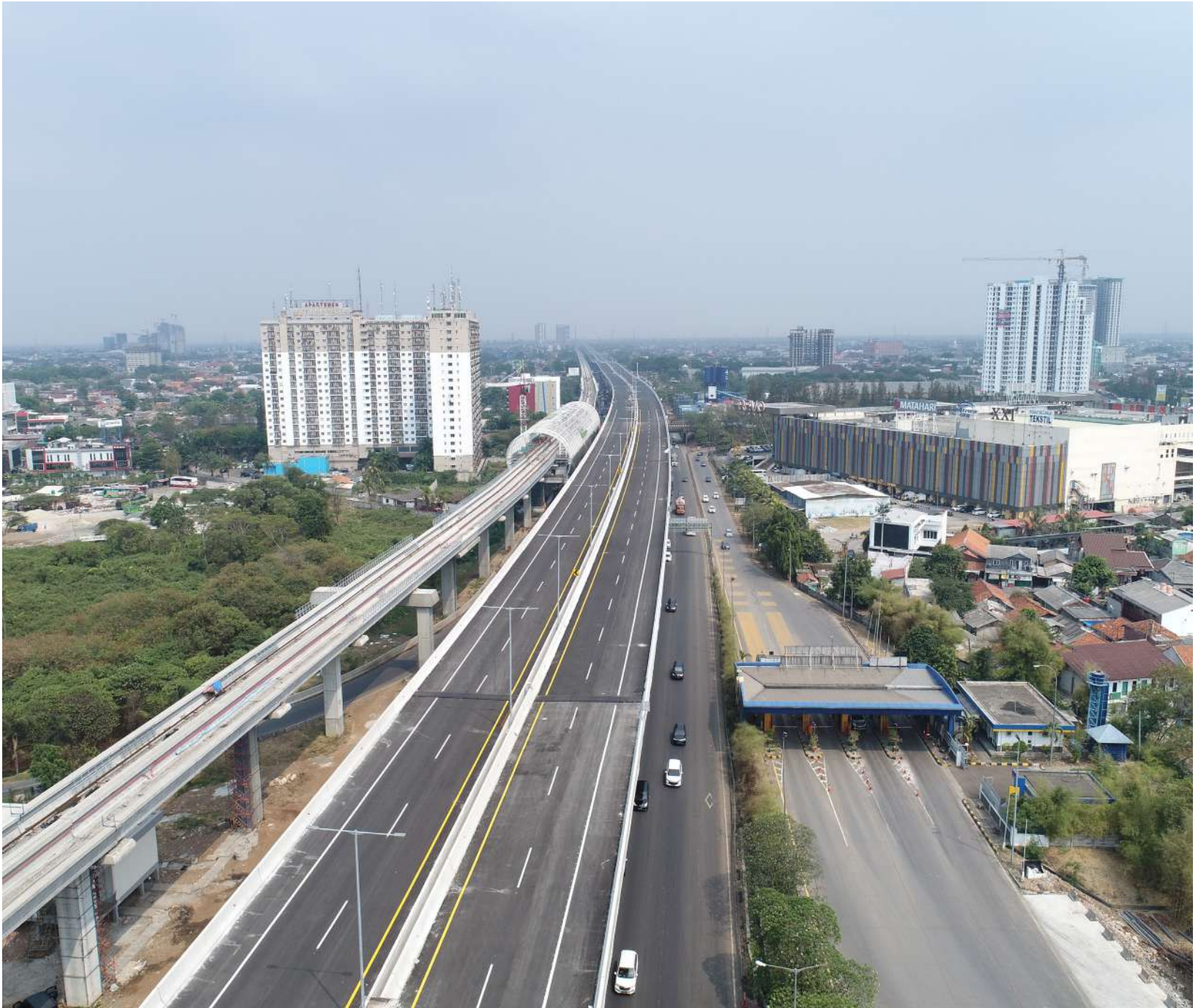
Jalan Tol Jakarta-Cikampek II (Elevated)
