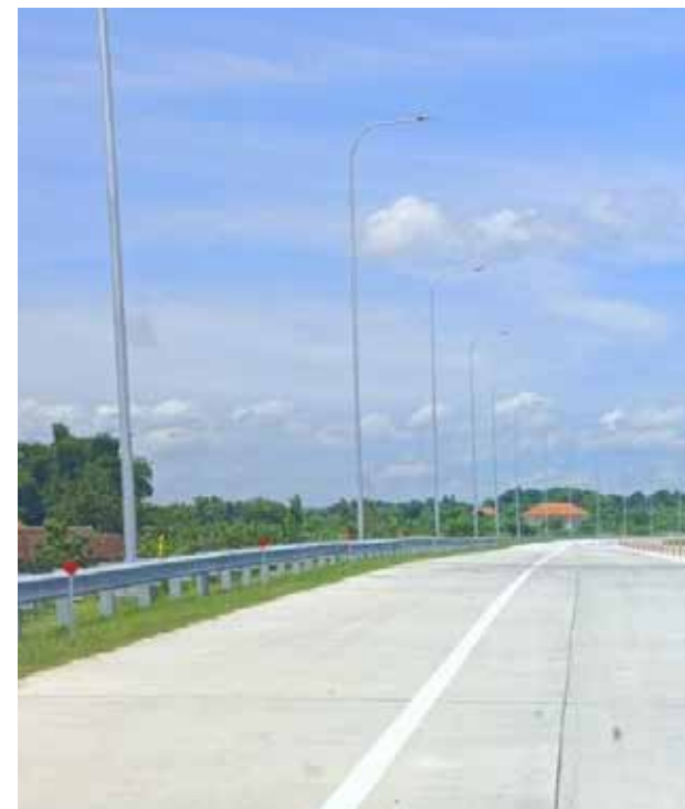
Pemasangan guardrail di Ramp 2 Junction Wringinanom Jalan Tol Krian-Legundi-Bunder-Manyar
